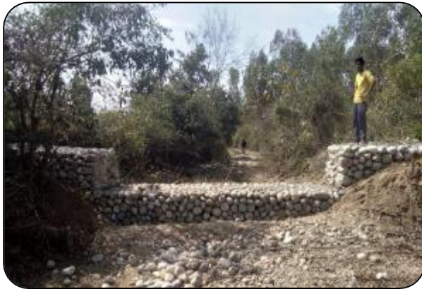
Gabion and Dyke
