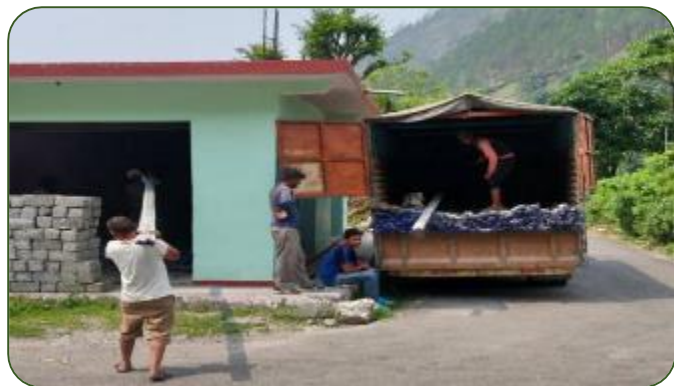
Transportation of pipes from store to Pindar valley
