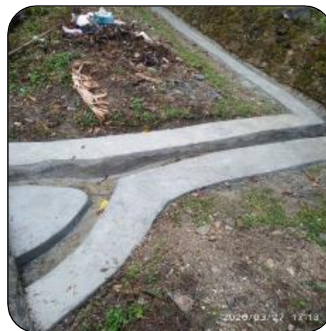
Construction of canal under EPA
