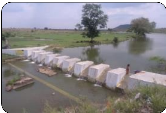
Stop dam reconstructed in Kalothara village
