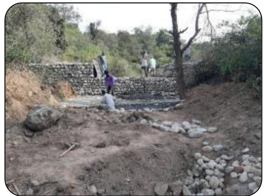
Construction of Gabion
