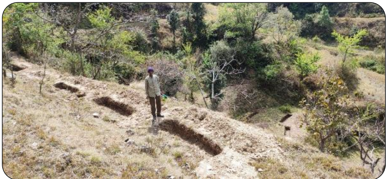
Trenches dug in Chanch Village, Almora
