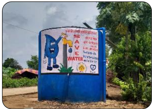
Drinking water supply system in Malpura village
