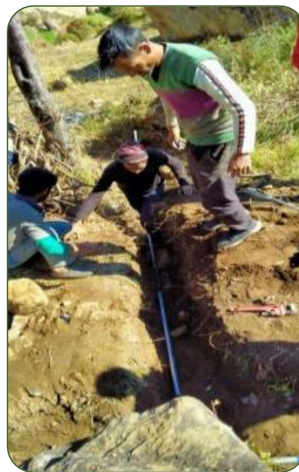
Laying out of pipes
